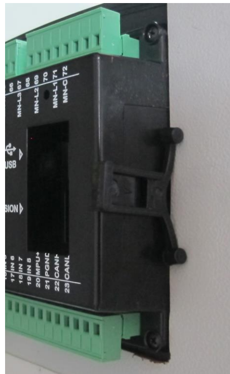
Installation of self retaining type bracket
